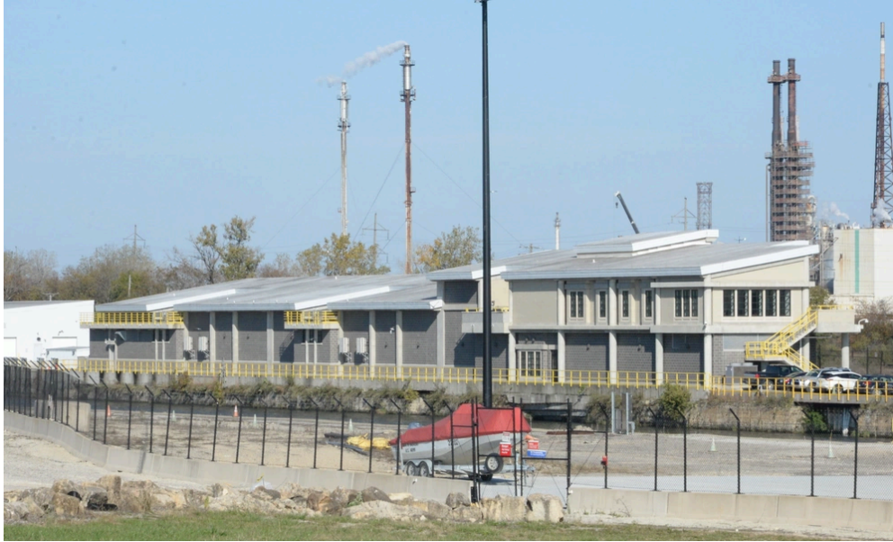
Figure 1 Electric Dispersal Barrier 1 Control Building, Romeoville, IL
