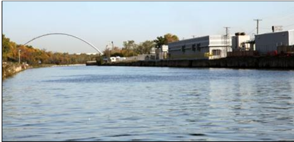
Aquatic nuisance species electrical dispersal barrier system, Romeoville, Illinois
